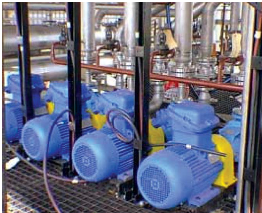
Fig. 1: Ex equipment must be suitable for the explosive environment.
